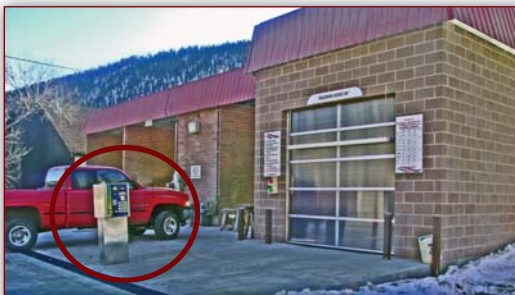
Entrance to car wash after remodel. Circled area shows the Unitec Wash Select II pay station.
