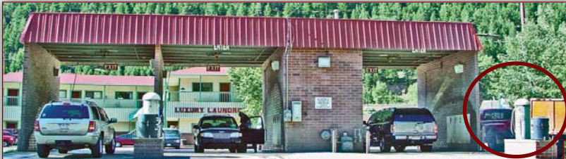
This is a shot of the car wash entrance before the remodel. Circled area shows where the automatic will be built.
