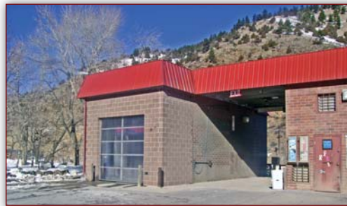
Exit side of the car wash after the remodel.
